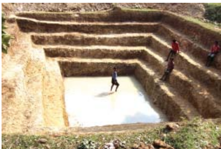
Excavation of tanks with 1:1 slope.
